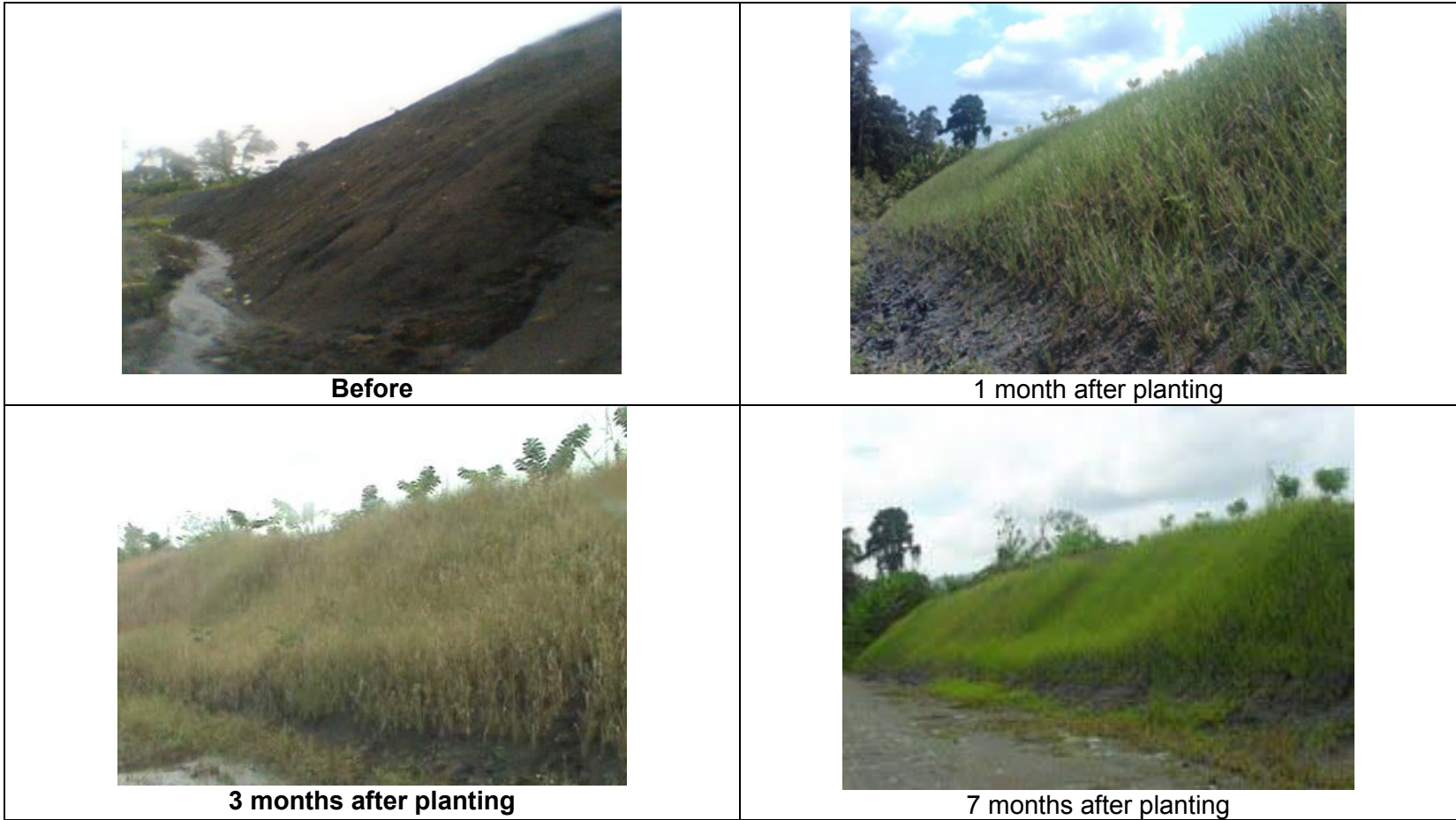
Figure 14: The Growth of Vetiver Grass on Slope of Yetti – Arso Road Link KM 106+750 s.d KM 107+100
