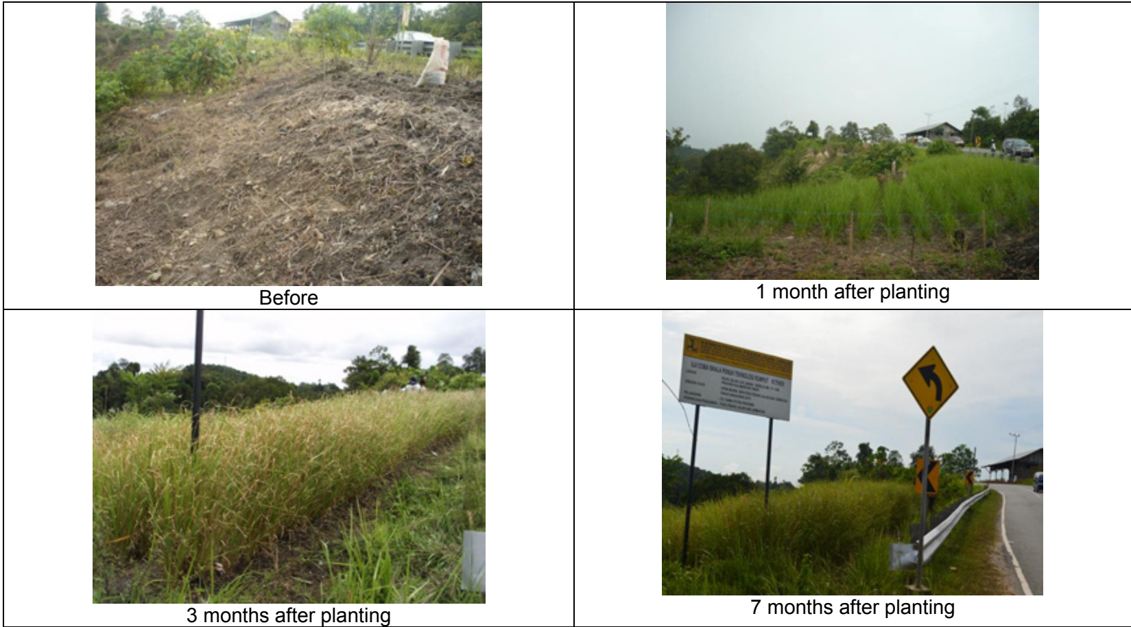
Gambar 12: The Growth of Vetiver Grass on Slope of Loa Janan – Gereja Road Link KM. 17+400 s.d 17+502, East Kalimantan
