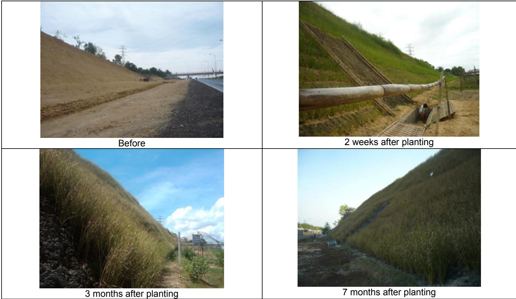
Gambar 10: The growth of vetiver grass on Slope of Surabaya – Madura road link Sta. 1+195 s.d Sta. 1+495
